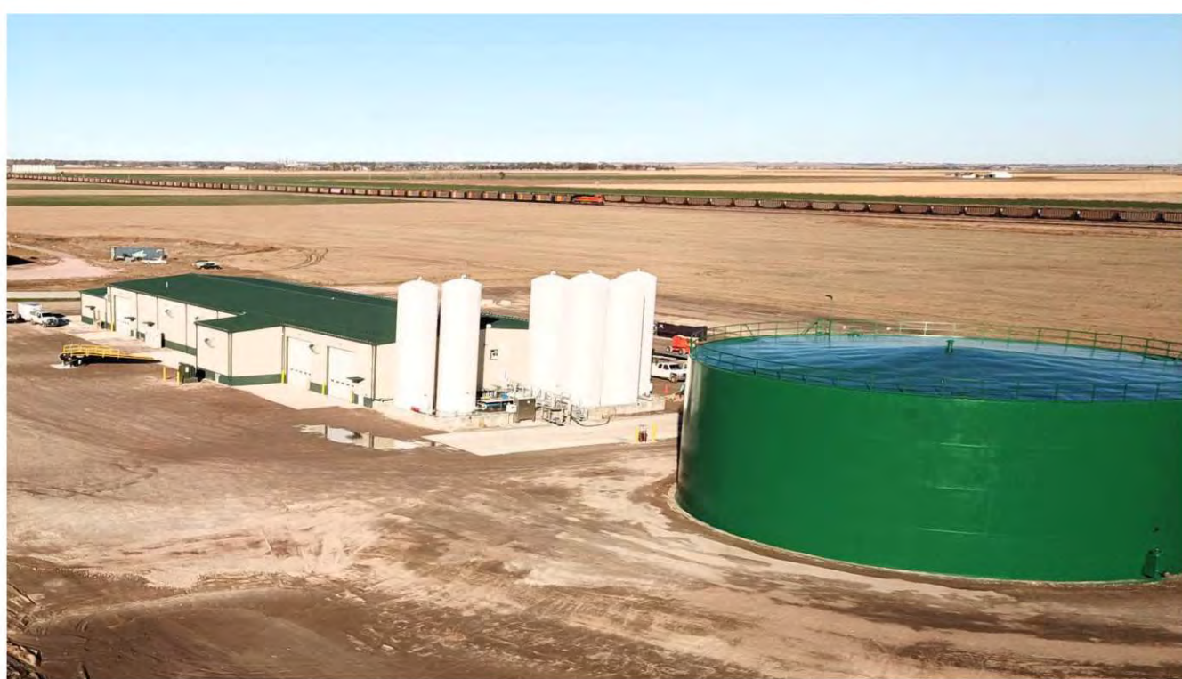
BULK TANK, LOAD PAD AND DIKE EXAMPLE
